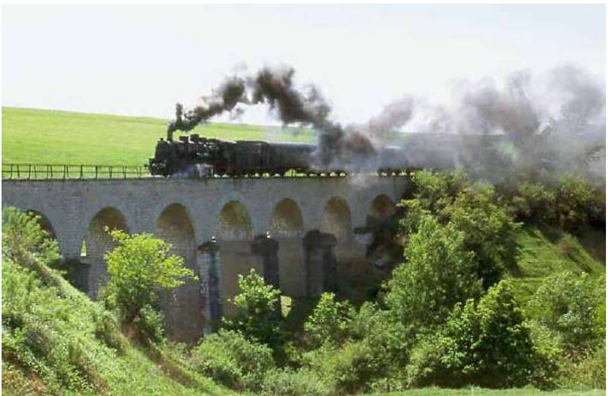
Fig.2 – A ponte Racovița
